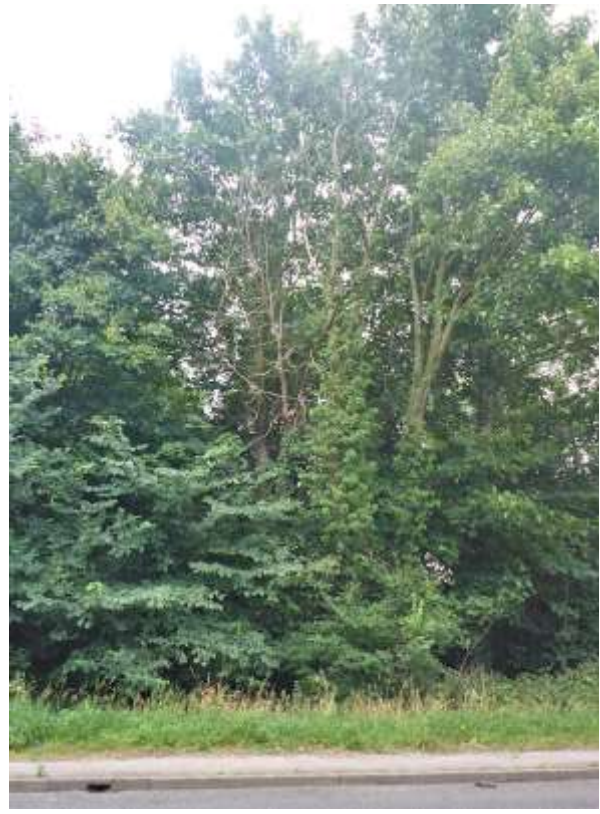
8. Fell dead elms within falling distance of road.
