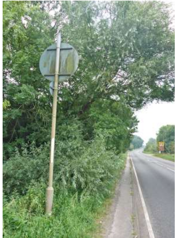
6. Cut back willow over road.
