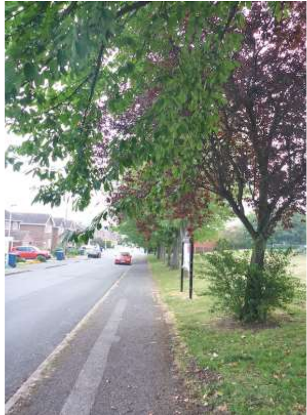
2. Crown lift over pavements & clear lights.
