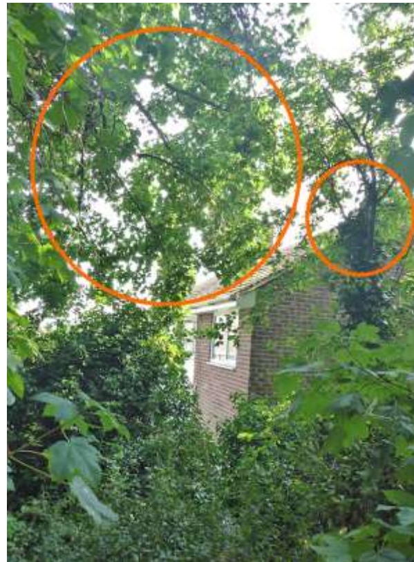
16. Cut back overhanging sycamore branch & damsons.
