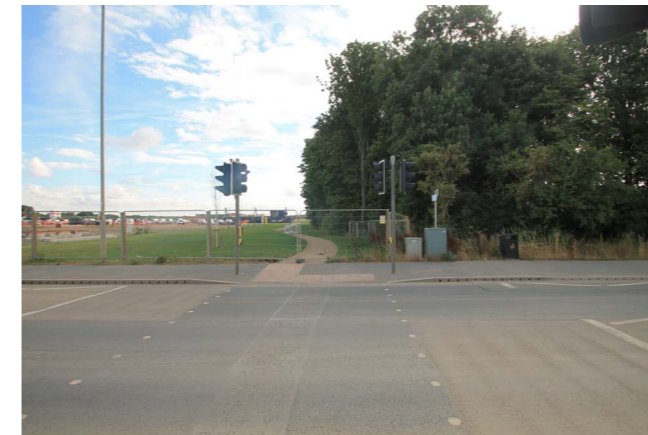
Pedestrian crossing already installed opposite access point to the site.
