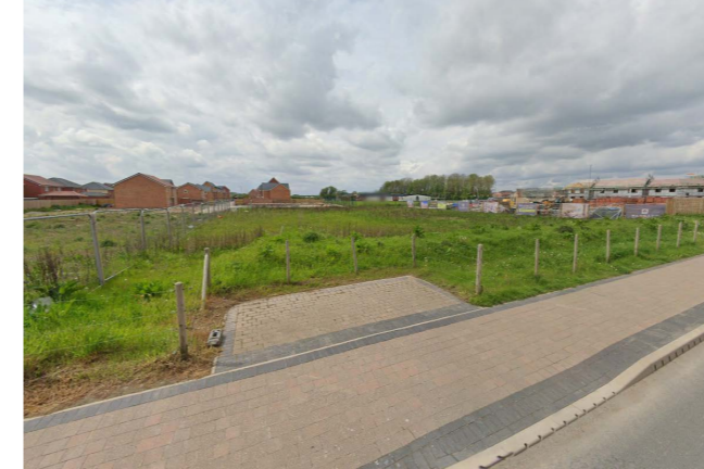
Clear site, ready for development.
