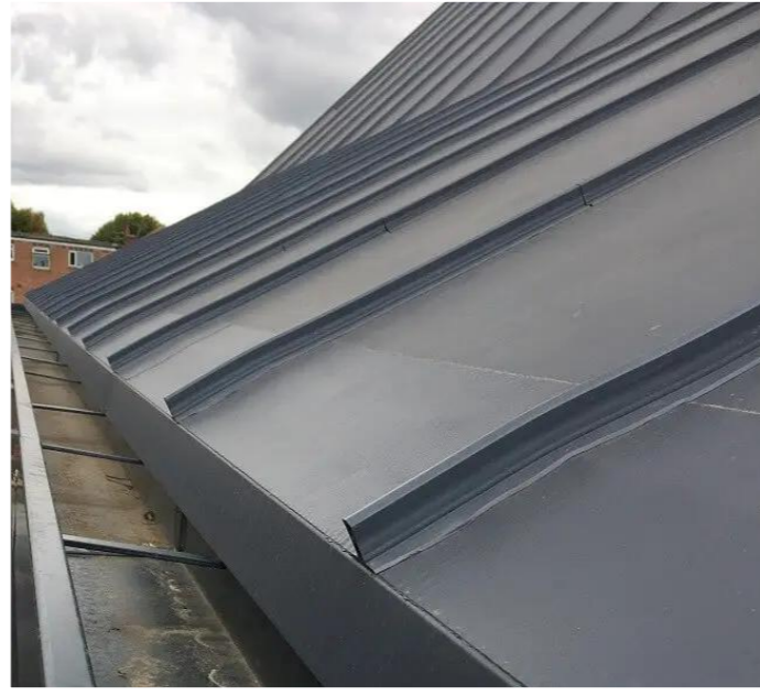
Single Ply Roof Membrane
